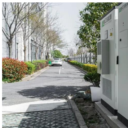
Off-grid photovoltaic folding container for aquaculture
